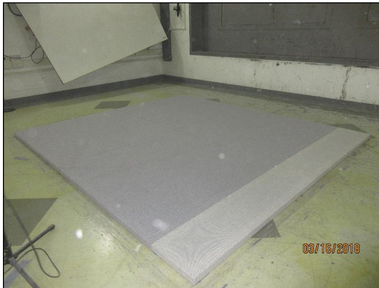
Photo No. 1 View of Installed Specimen
